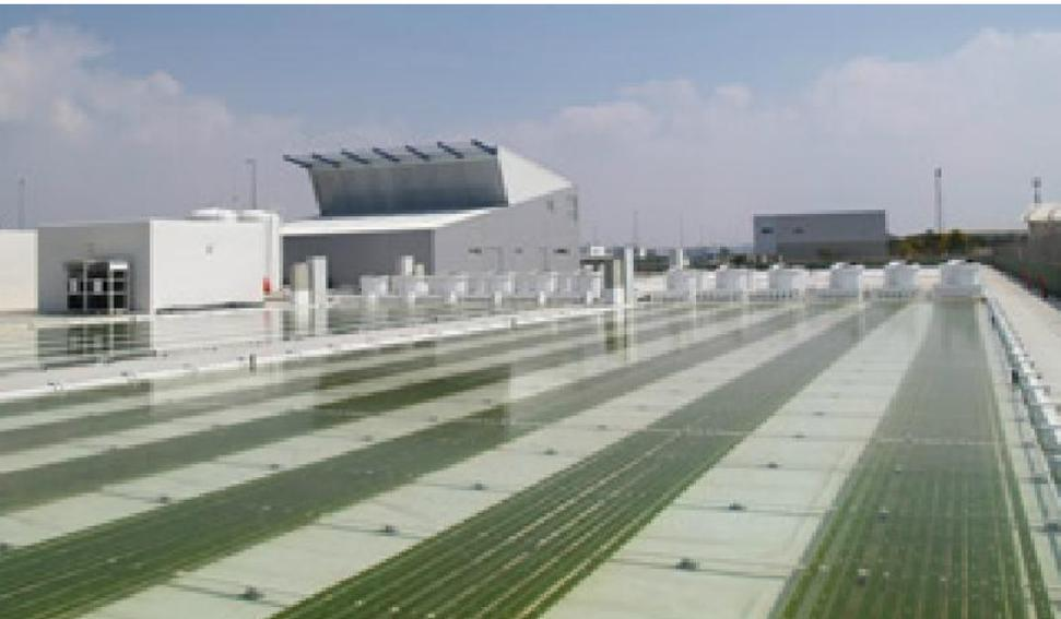
They developed an unique microalgae production system based on photobioreactors. This patented system consists of a number of outdoor closed photobioreactor. These closed photobioreactors prevent any type of contaminants entering the system and in this way they provide high quality microalgae. The systems are monitored and automated, which avoids direct manipulation during harvesting and reduces contamination risks.
